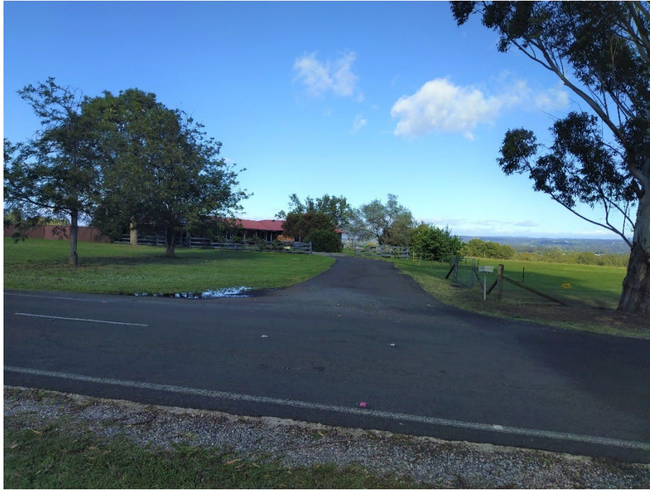
Figure 2 – Photograph 9: Convent Precinct viewed from Macquarie Grove Road entrance
