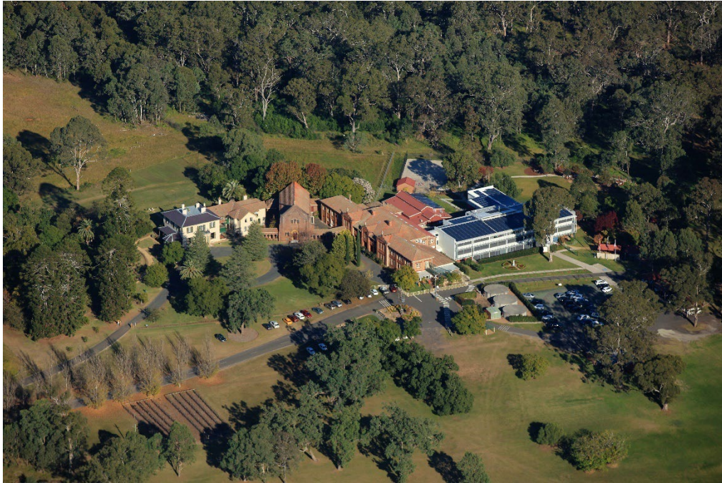
Figure 2 – Photograph 1: Aerial photograph extract of the Mater Dei School and Wivenhoe Precinct
