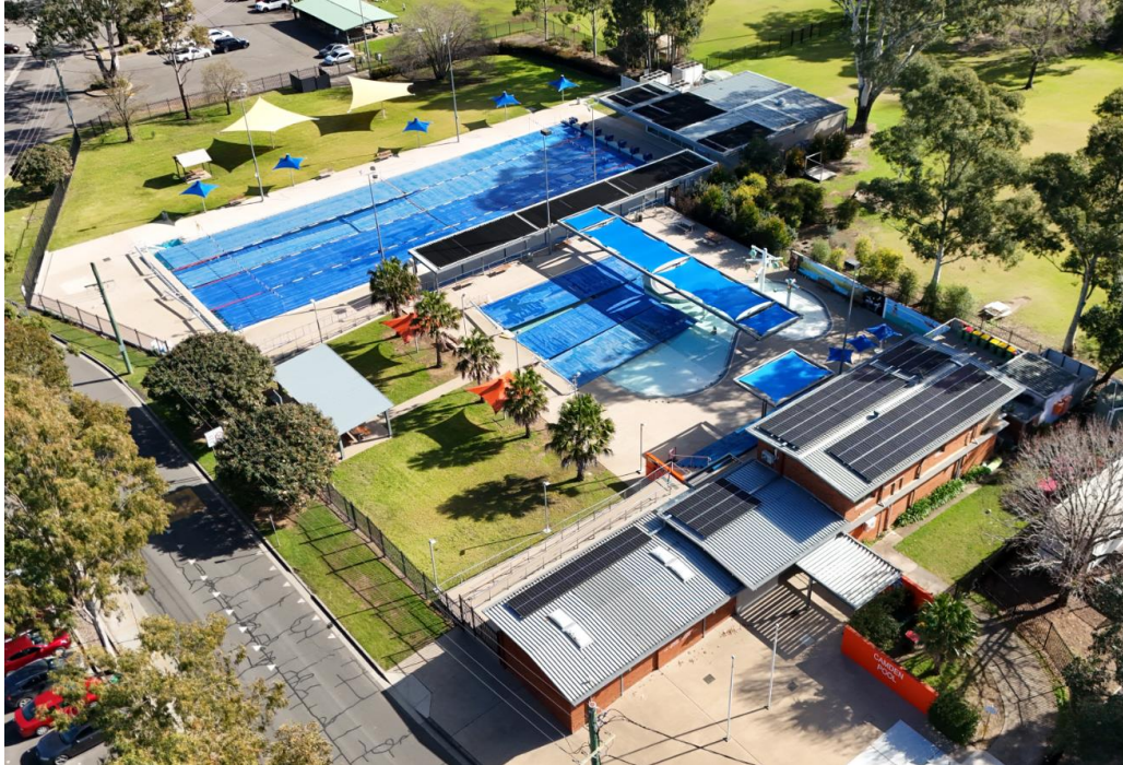
Installation of a 28.16kW rooftop solar system at Camden War Memorial Pool, bringing total capacity to over 500kW across 11 sites with more on the way. Location and extent of panels was restricted by heritage zoning within the Camden township.
