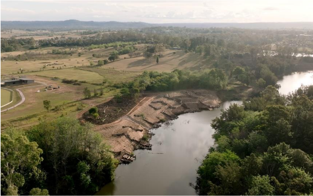
Aerial photo of in progress restoration works along a 300m section of the Nepean River at Ferguson Land showing installation of 8 engineered log jam structures completed in partnership with Sydney Water in October 2023 to provide enhanced resilience to future flooding events and prevent soil loss.
