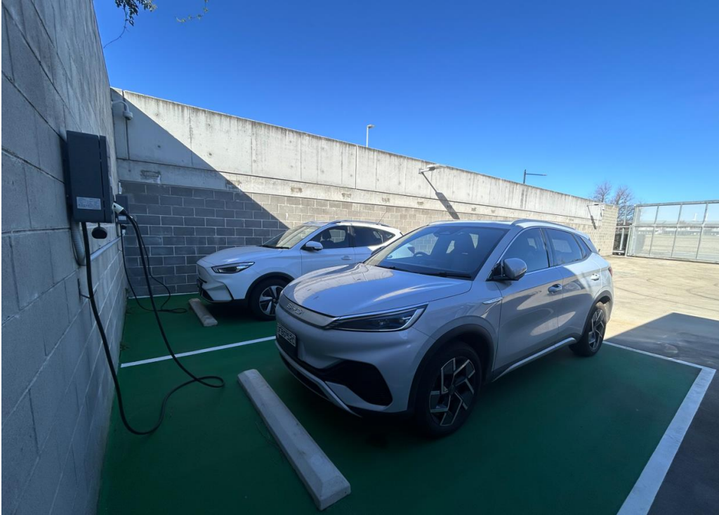
Council staff pool vehicles charging at the Oran Park Administration Building including a BYD Atto and MG Essence.
