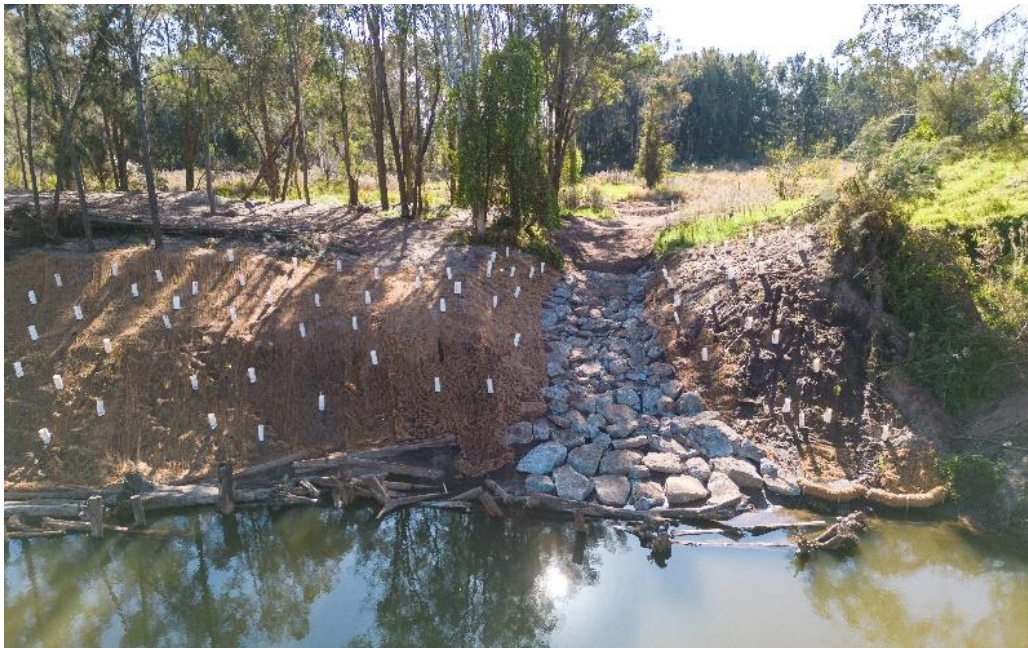
Bank restoration works were completed at Spring Farm showing log jam fish habitat, restoration planting and erosion protection measures.
