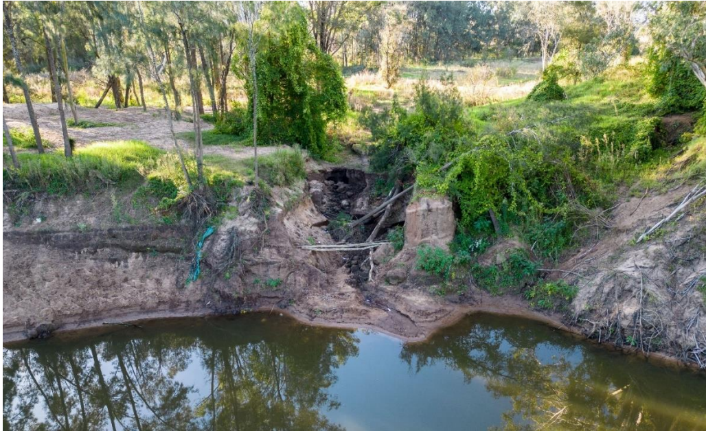
Photo of erosion scour and Nepean River bank from flooding events at Spring Farm prior to restoration works being undertaken.
