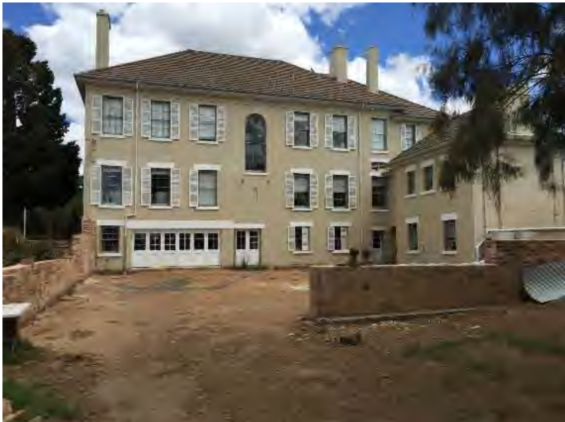
Figure 69: Current Oct 2017 view of the rear (north elevation) of the property. Note the rear courtyard brick wall had gone past the safe lean point and had been assessed by a structural engineer as unsafe and had to be carefully dismantled for safety reasons. TTA Oct 2017
