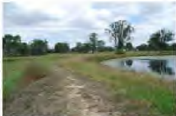
Plate 4. View south across dam wall
