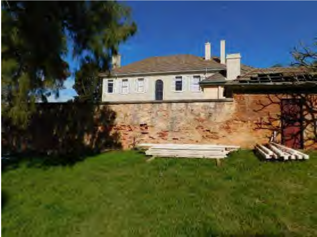
Figure 68: The rear brick wall surrounding Oran Park House showing its poor condition. TTA 2013
