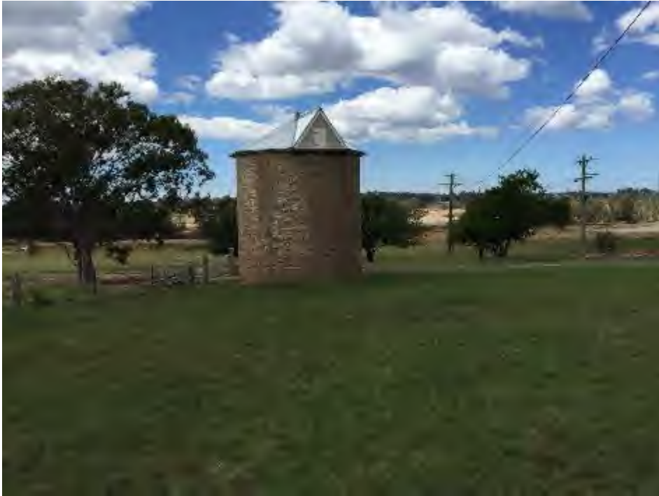
Figure 92: Silo looking east. TTA Oct 2017
