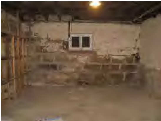
Figure 76: Cellar, Basement level, looking west. TTA 2013
