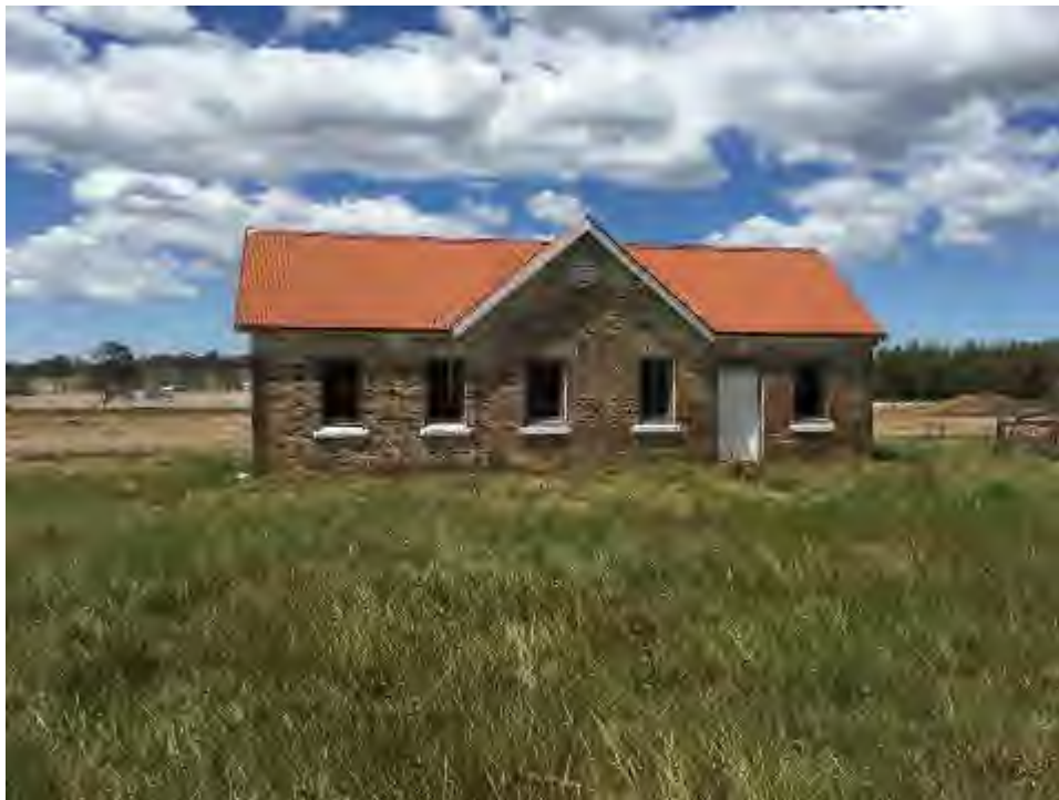
Figure 81: Coach House, west elevation. TTA Oct 2017
