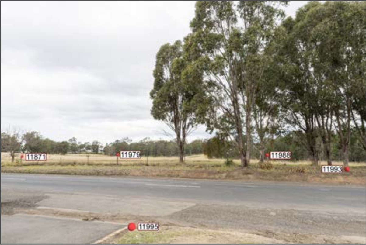
ORIGINAL PHOTOGRAPH INCLUDING SURVEYED ALIGNMENT DATA
