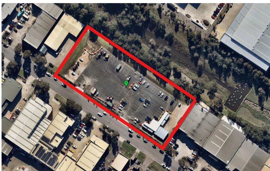
Figure 1: Aerial Photo – 55 Topham Road Smeaton Grange
